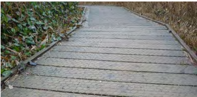
Boardwalks have netting cover and a low kick board to edge
