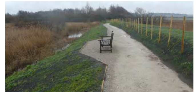
Main footpath to beach along western side of reserve has been recently upgraded
