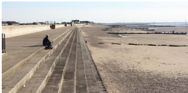
At some points the steps down allow access straight onto the beach
