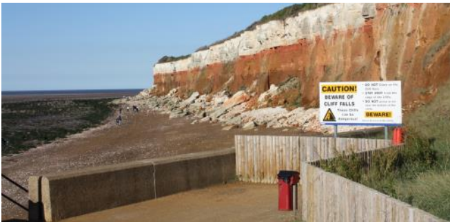
Access down to the base of the cliffs is limited to steps only
