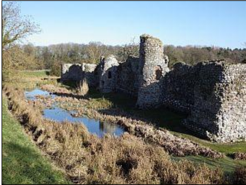
The moat and pond at Baconsthorpe Castle are supplied with spring water.
