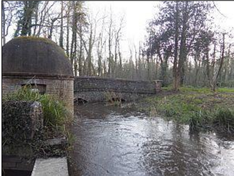
The River Glaven at Bayfield Bridge. The building on the left houses a Victorian hydraulic ram machine which once supplied Bayfield Hall.
